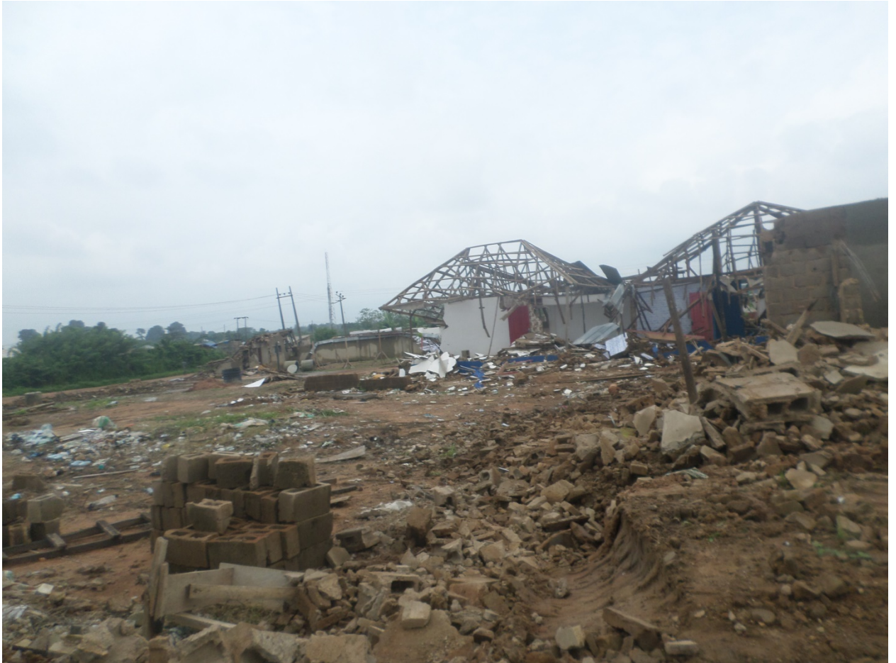
Figure 10: Plate showing demolished buildings at Fashade in Ajoda New Town
