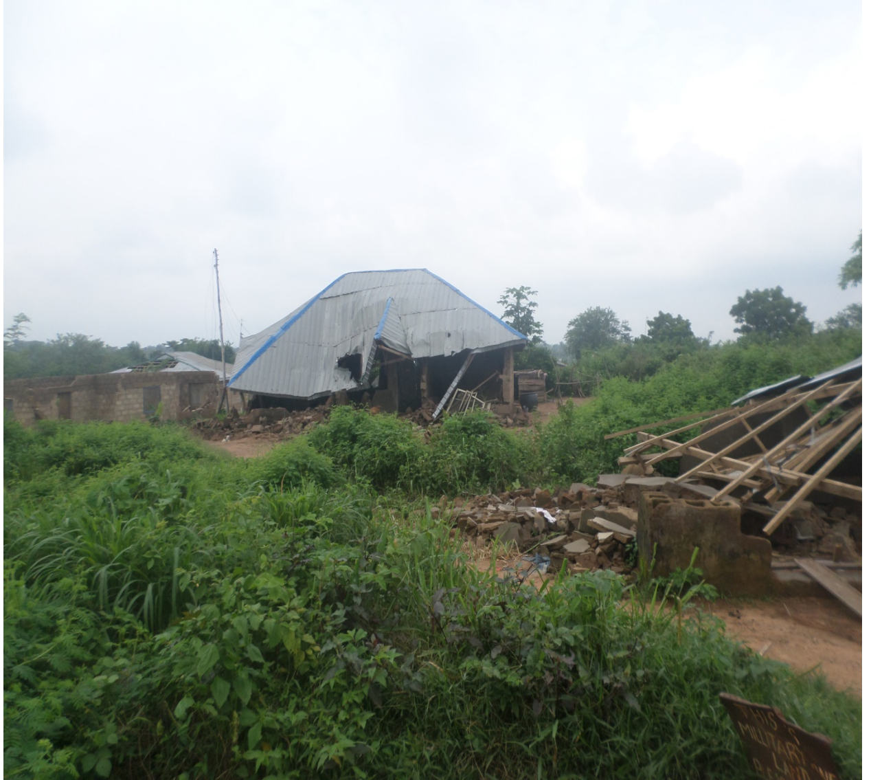
Figure 11: Plate showing demolished buildings at Ajule in Ajoda New -Town
