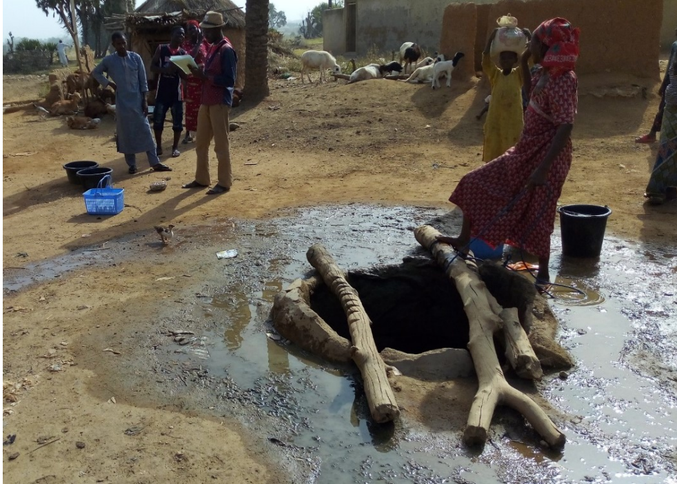
Plate 4.1. An unprotected hand dug well in the Bauchi-Alkaleri-Kirfi area.
