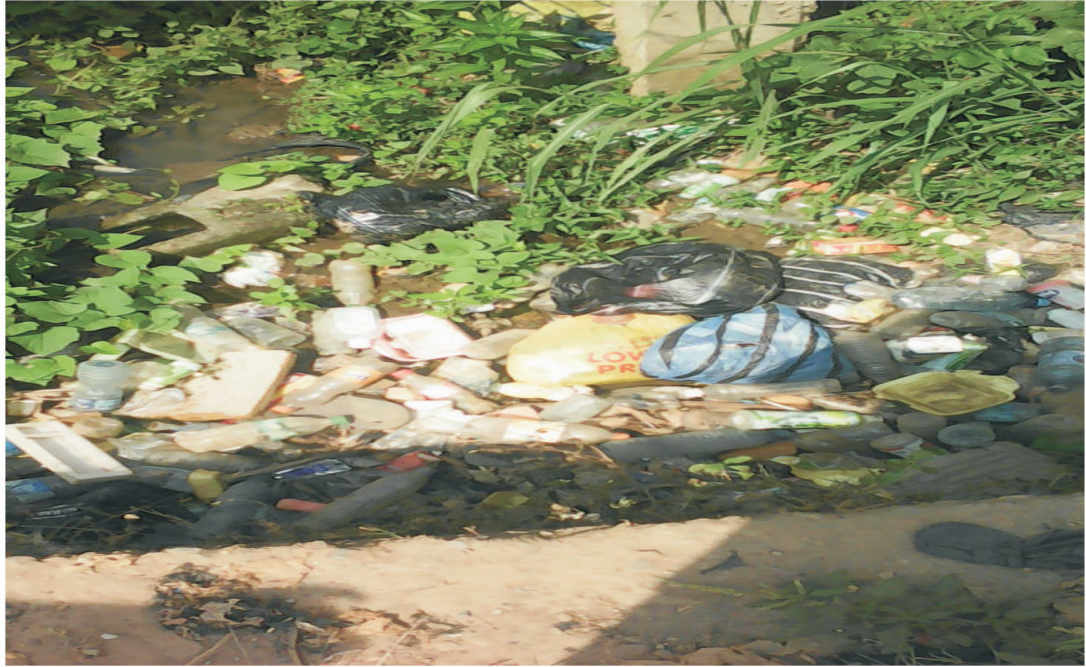
Refuse Dumped Inside a Drainage, Along Yemetu Area, Ib.
