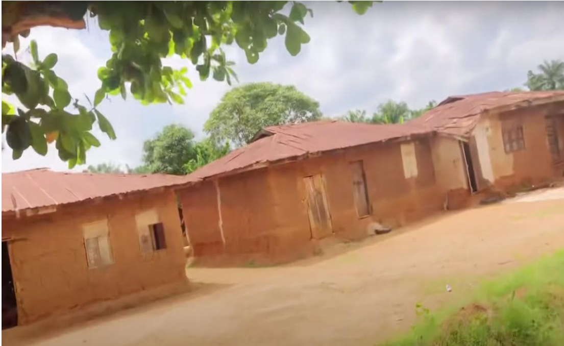
Plate 4.20: Row of houses in Igbo Olodumare, the village closest to Igbo Olodumare Sacred Grove. Source: Field Survey, 2019
