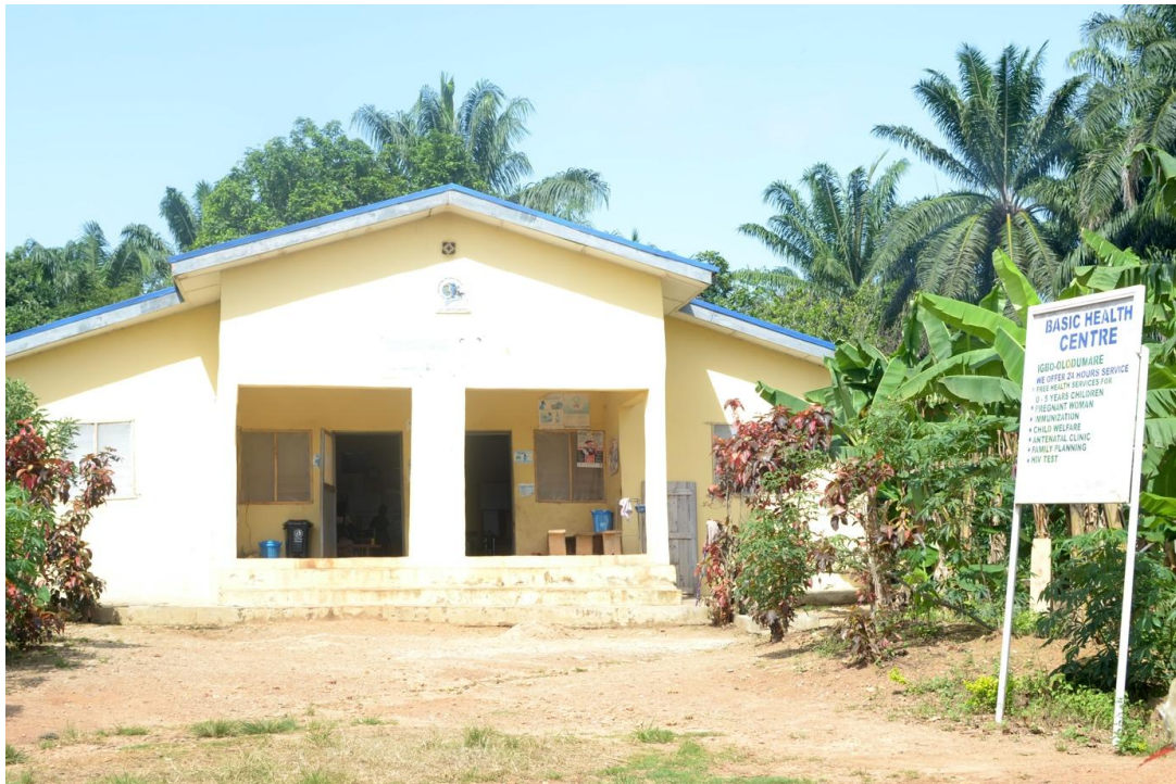
Plate 4.19: Front view of the Basic Health Centre in Igbo Olodumare Source: Field survey, 2018.
