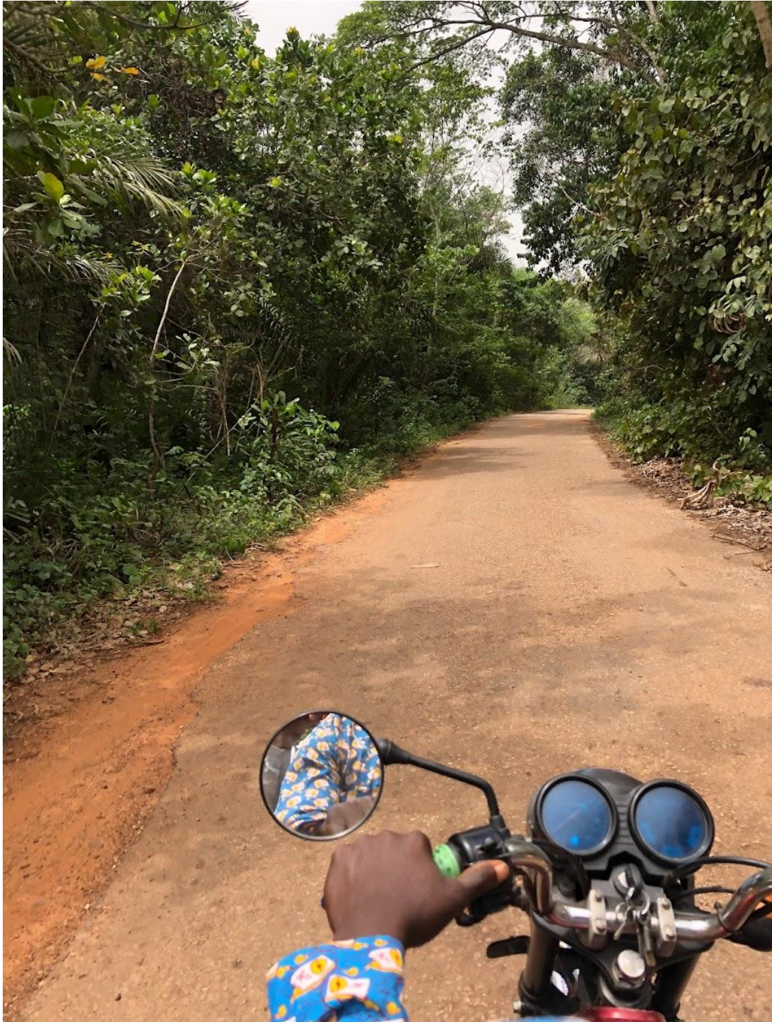
Plate 4.2: The best section of the road to Igbo Olodumare from Oke-Igbo, showing remnants of the old tar which has completely washed off in most other parts. Source: Field survey, 2019.
