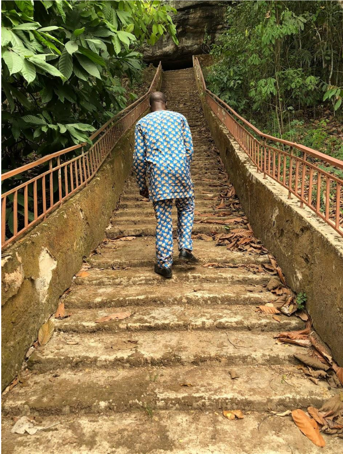
Plate 4.10: Stairways to Oke-langbodo. Source: Field Survey, 2019
