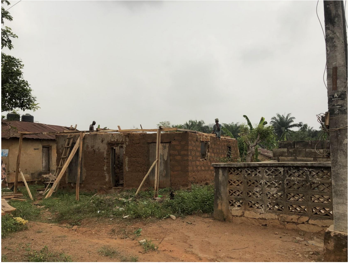
Plate 4.3: A mud house under construction in Igbo Olodumare. Source: Field survey, 2019.
