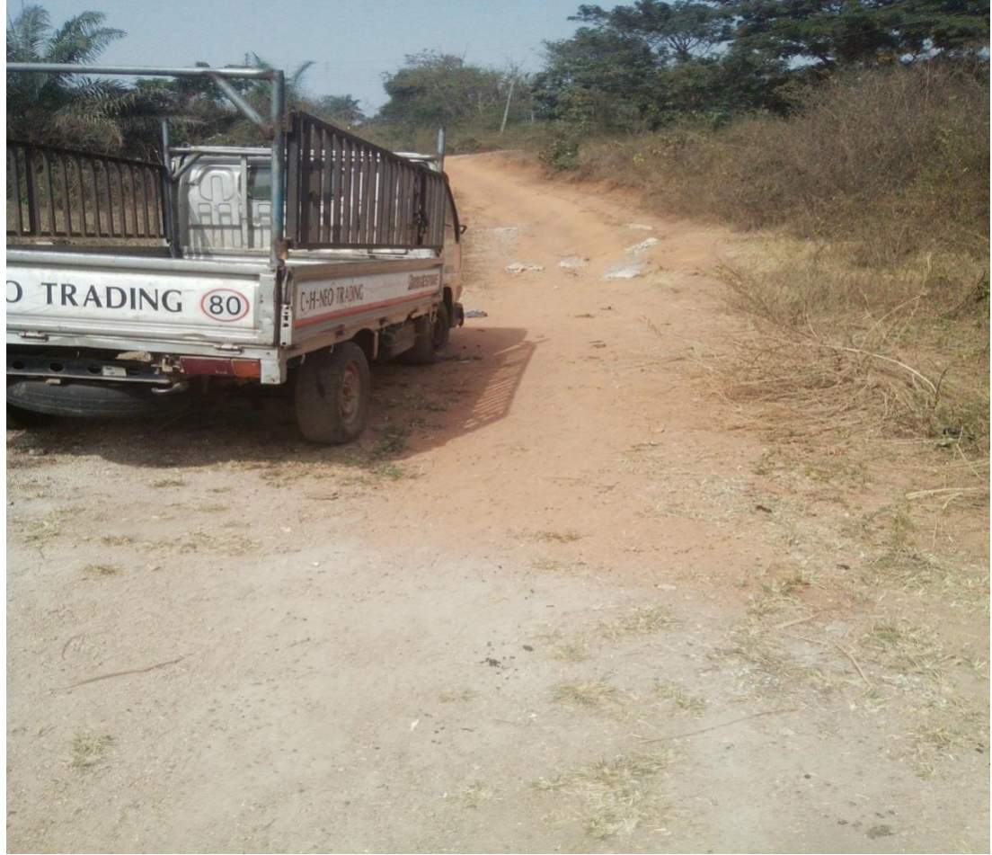
Figure 4.20: State of roads in Ondo West rural areas
